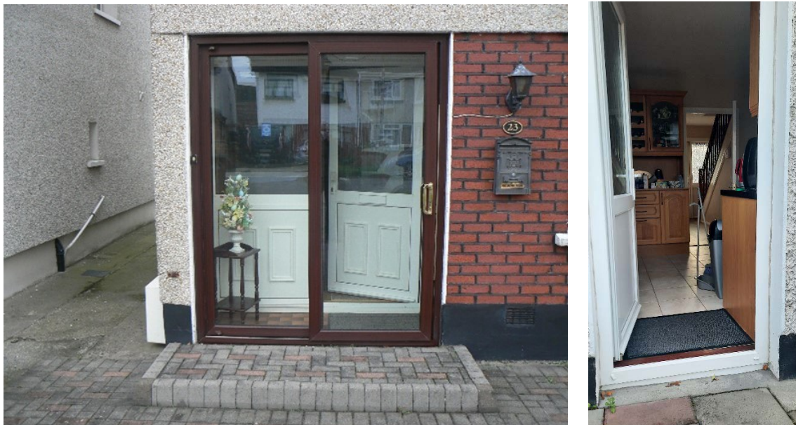
Figure 8 - Stepped access at both front and rear entrances
