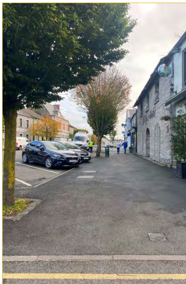
Resurfaced path in the town centre
