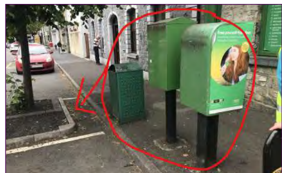
Example of utility boxes located on footpath where alternative space was available.
