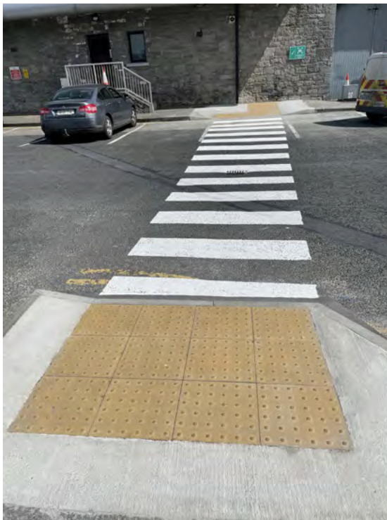
► Two newly installed tactile paving pedestrian crossing points
