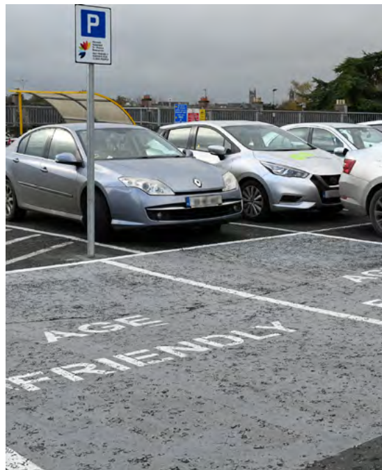
► Installation of two Age Friendly Car Parking Spaces
