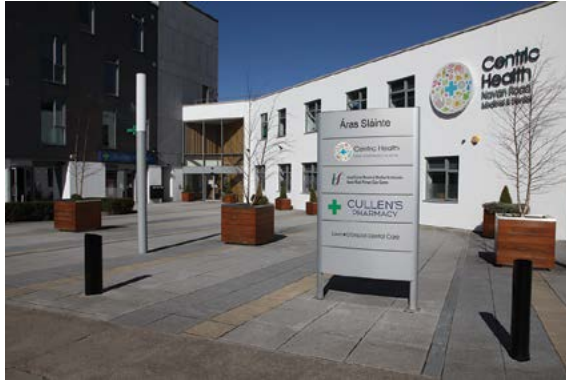
Navan Road Primary Care Centre
